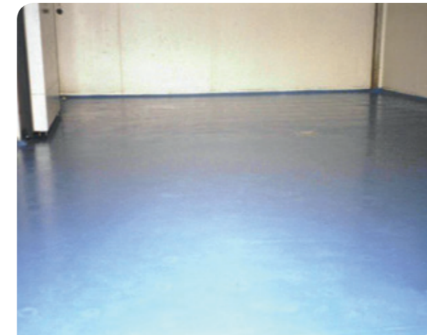
Picture 2: Thioplast™ EPS coating of the floor in a slaughterhouse
