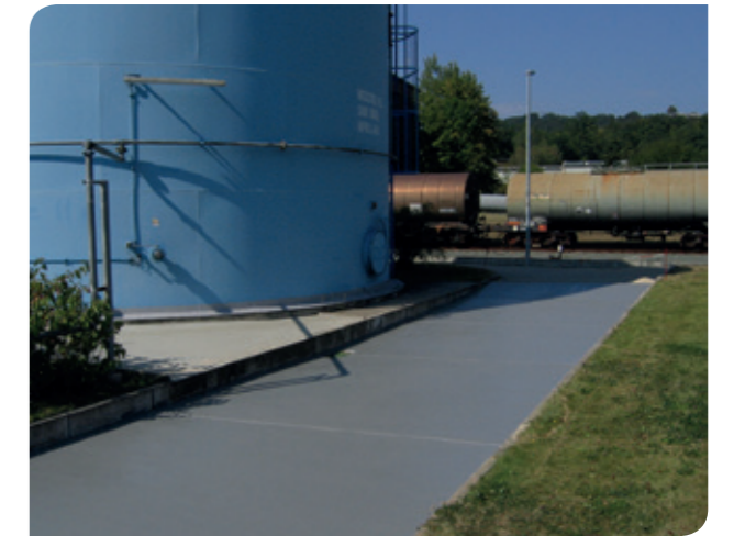
Picture 3: Polysulfide based joint sealant as a crack-bridging, chemically resistant coating
